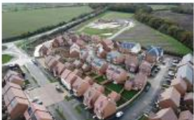
Whitstable Heights Working with Hyde we are developing 400 new homes, allotments and extension to a local nature reserve.
